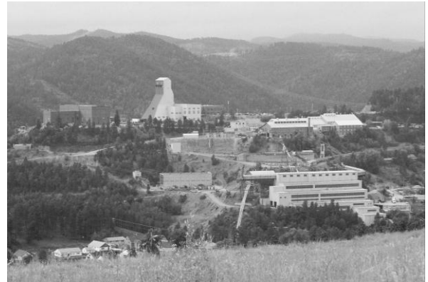
Figure 16. Yates shaft headframe and Homestake mine processing facilities.
