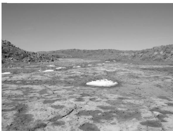
Figure 13. Present floor of an abandoned mine on Bluff H, about 1.5 miles east of the Riley Pass mines. The flat-lying stratigraphy has resulted in broad open floors at the base of the mining.
