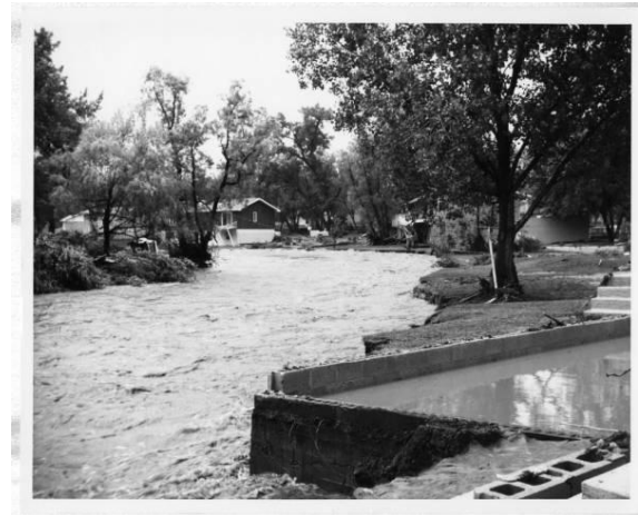
Figure 12. The destruction from the 1972 flood from Rapid Creek just upstream from Rapid City is evident by the foundations of former homes. This photograph was taken by the U.S. Department of Agriculture shortly after the destructive flash flood.
