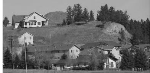
Figure 13. Several homes are built on top of massive gypsum beds in this area. Many additional areas of gypsum outcrop are evident. Homes at base of hill encountered scattered gypsum boulders while being built. Once the foundation has been constructed, it is imperative that water routing is maintained away from the foundation so as not to weather potential underlying gypsum stringers.
