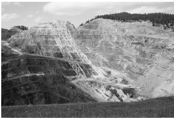
Figure 18. Homestake Mine Open Cut with Tertiary rhyolite dikes.
