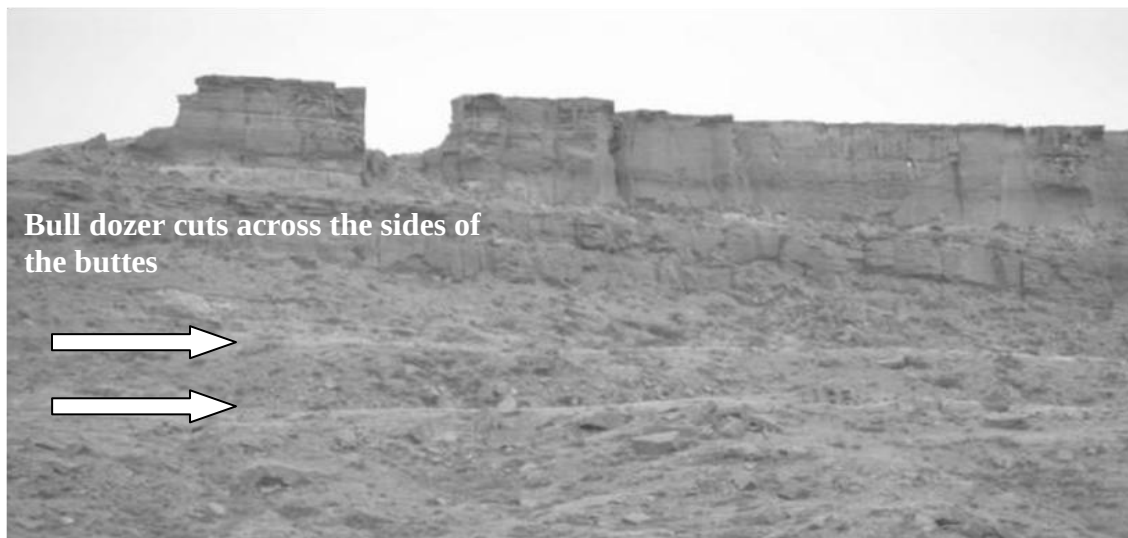
Figure 7. Bull doze cuts across the sides of the buttes below the Ludlow (bottom) and Tongue River (sandstone cliffs at top) contact. These were in an attempt to uncover lignite units that were the host for the uranium.
