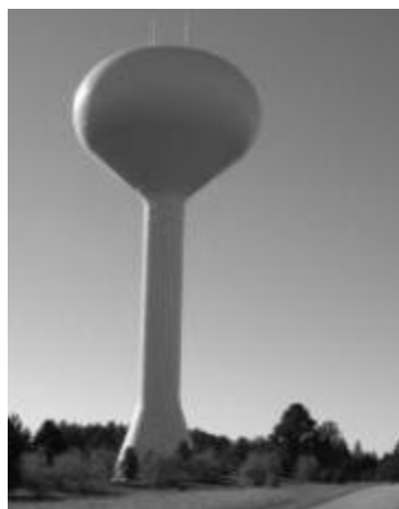
Figure 6. Rapid City's 'Ultra-High' 1 million gallon storage tank located across US Highway 16 from Stop No. 2.
