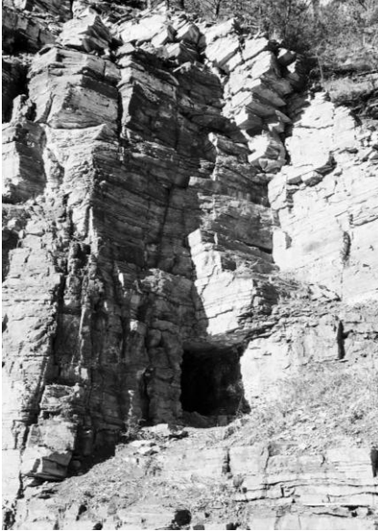
Figure 28. Adit following an intraformational conglomerate bed in the Deadwood Formation.
